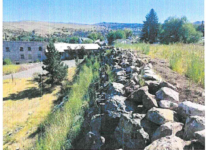
Photograph 8: Looking northeast along west leg of boulder retaining wall.
