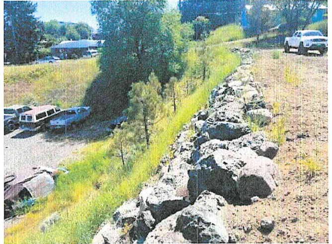
Photograph 6: Looking east along east leg of boulder retaining wall.
