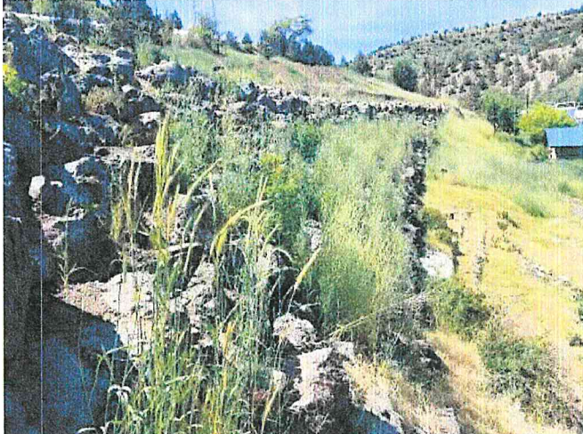
Photograph 7: Looking southwest along base of west leg of boulder retaining wall.
