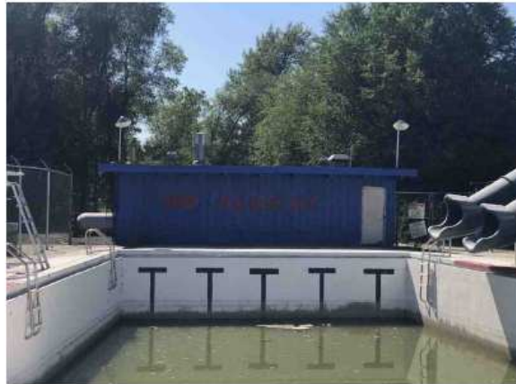
Pool Mechanical Building
