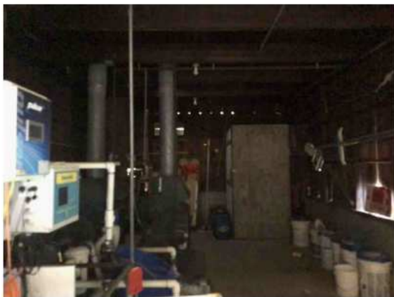
Interior of Mechanical Building
