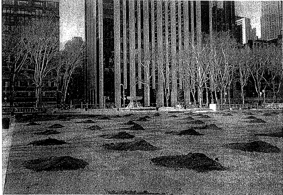
Use of biosolids on parkland in Manhattan, New York. Biosolids compost is piled on barren site to be spread for soil conditioning.
