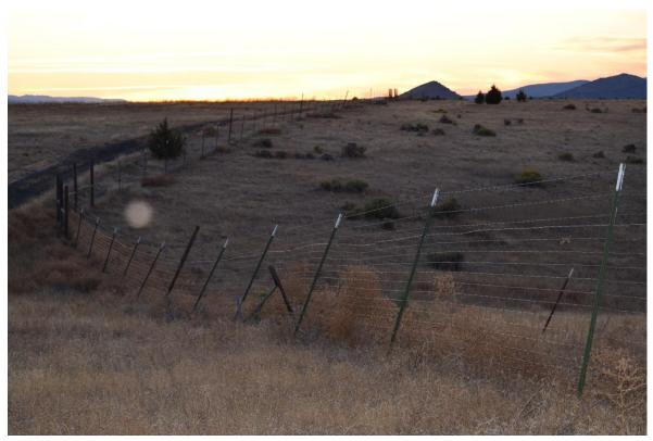
Figure 6: Large Areas of Perimeter Fence are Leaning (Kestrel, LLC).
