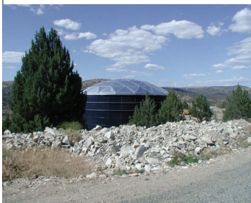
Reservoir No. 6 located on La Costa Road west of John Day.
