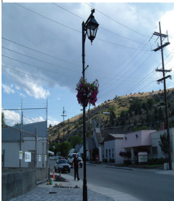
New light poles with hanging baskets brightens up SE Dayton Street.
