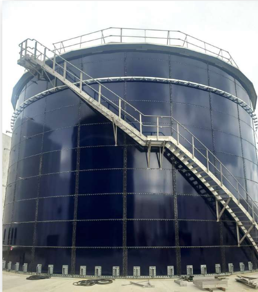
Above photo: 1 Million USG EVERSTORE® Glass Fused-to-Steel Tank with Spiral Staircase
