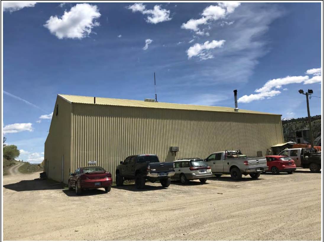
View east of the main shop building.
