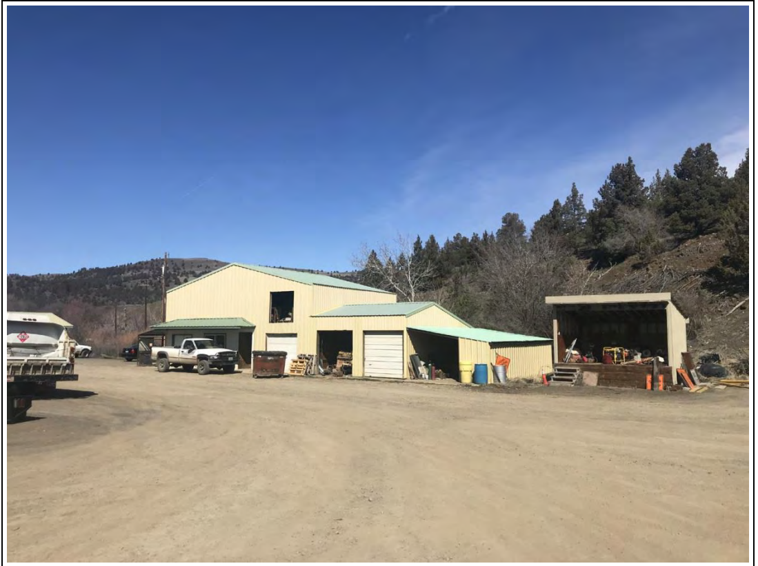
View northwest of the secondary shop building.
