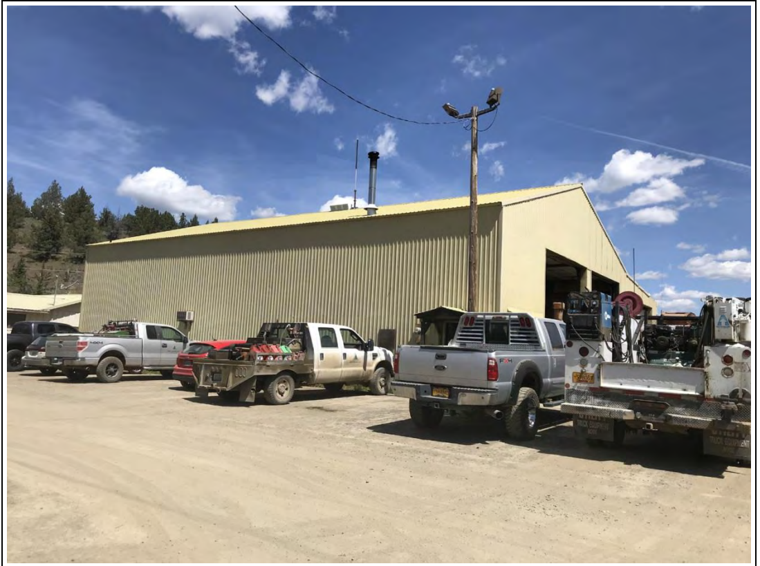
View northeast of the main shop building.
