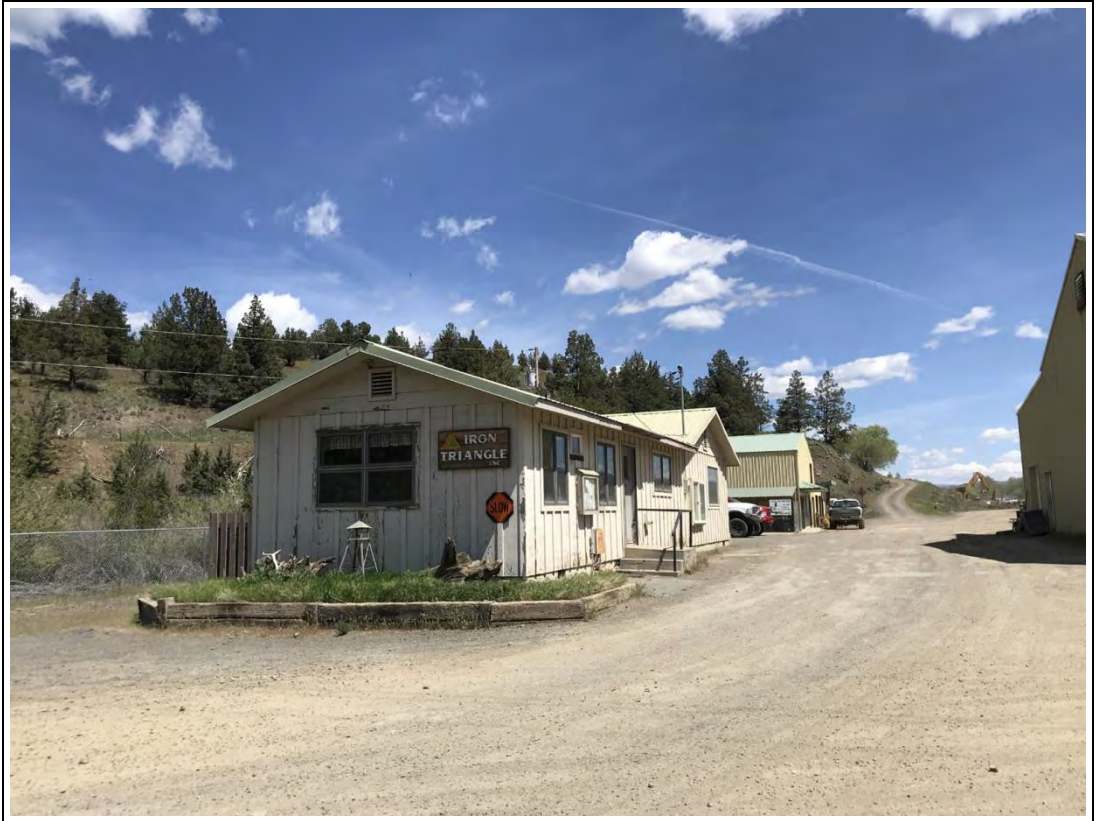
View east of the office building.
