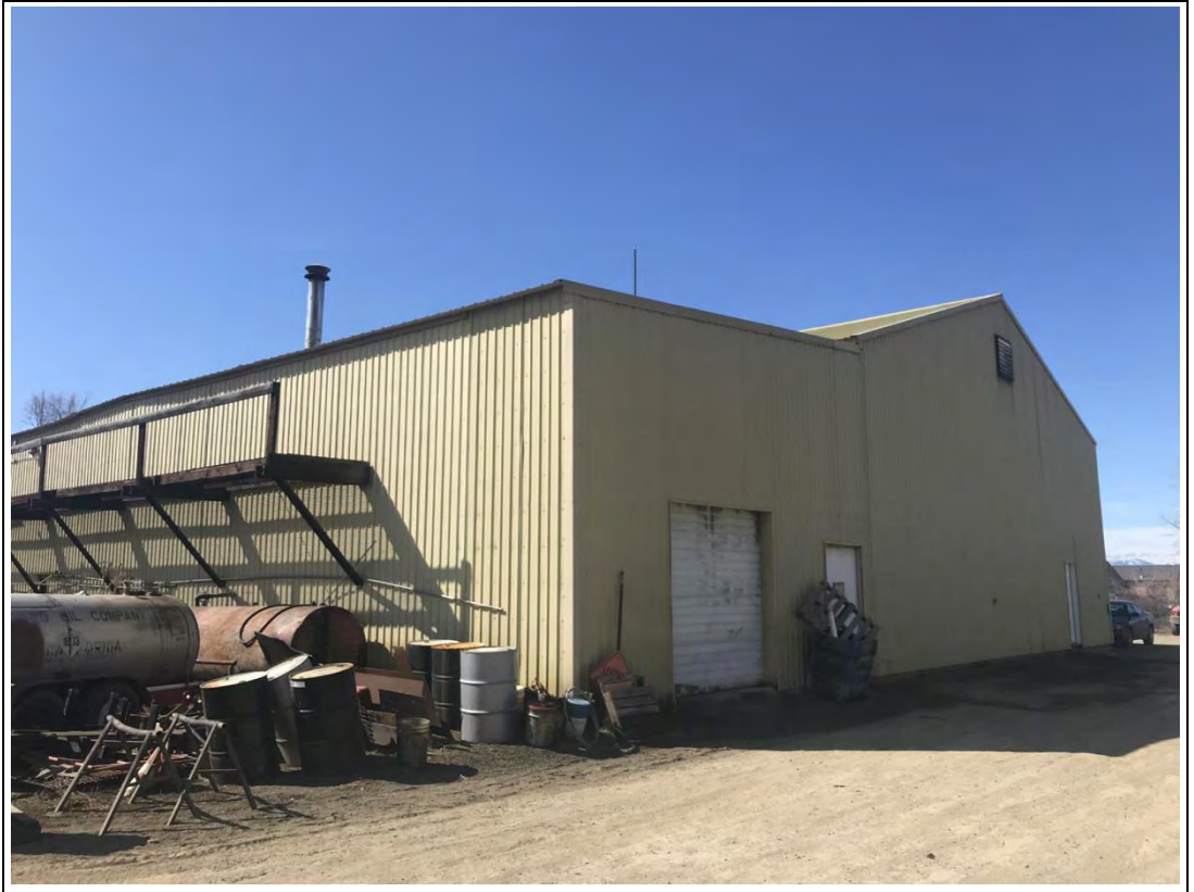
View southwest of the main shop building.
