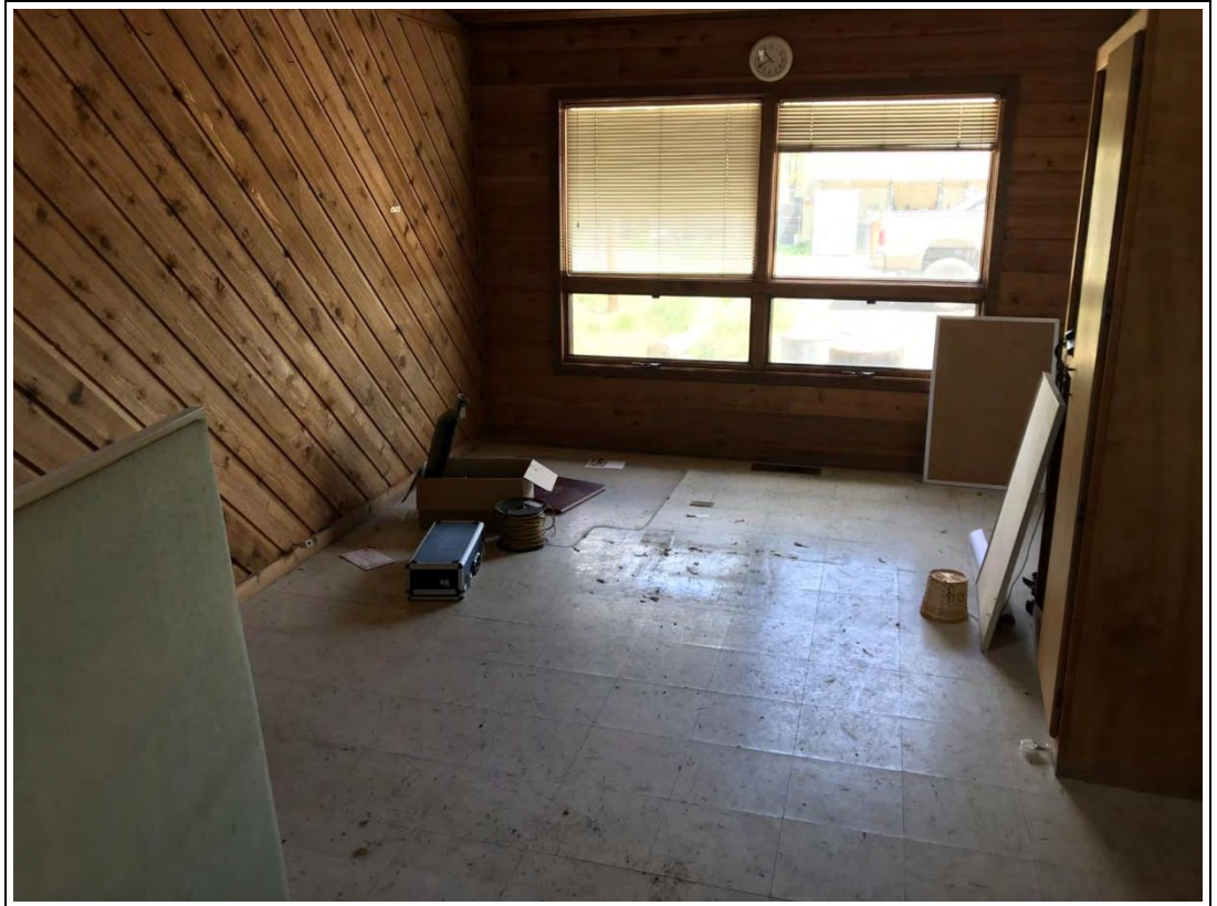
Interior of the office building.
