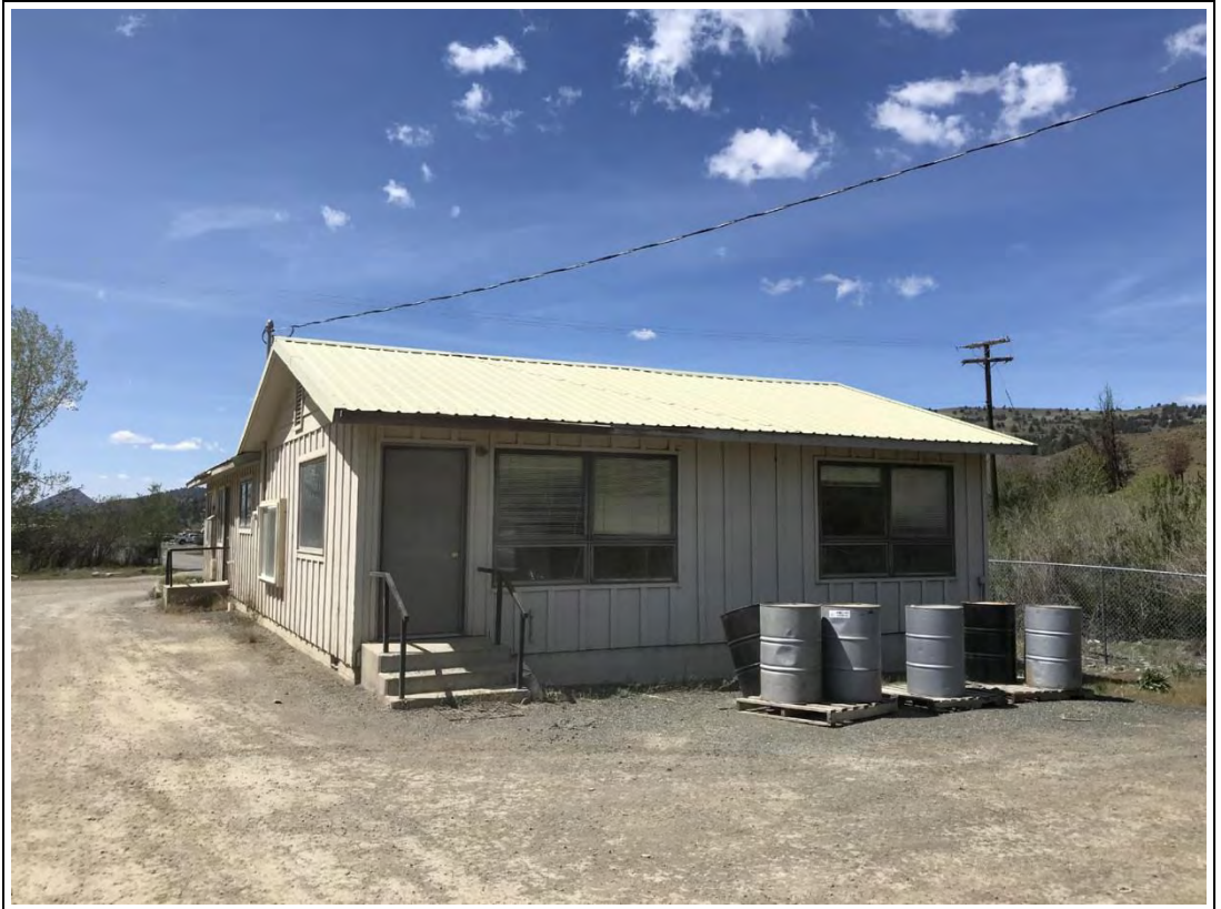
View west of the office building.
