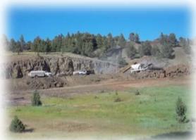
GRANT CO. ROAD DEPT. ROCK CRUSHING
