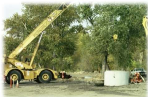
LIFT STATION CONSTRUCTION AT COUNTY ROAD DEPARTMENT SITE
