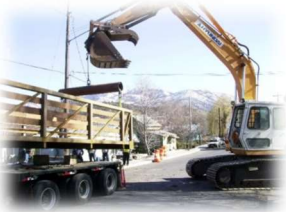
BRIDGE ST. PEDESTIAN BRIDGE INSTALLATION
