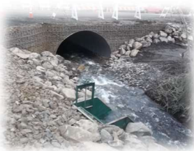
VANCE CREEK CULVERT
