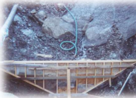
CANYON CITY SPRING BOX CONSTRUCTION
