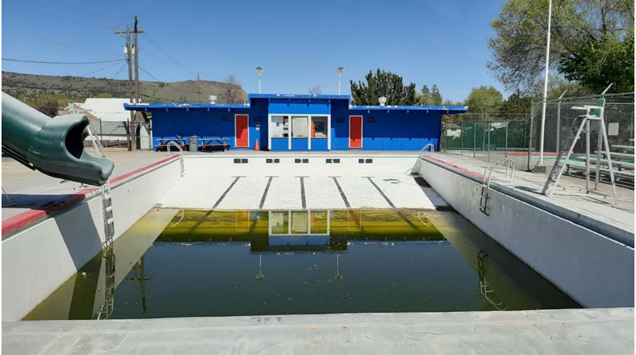
Figure 9. Pool and deck looking east toward the pool house
