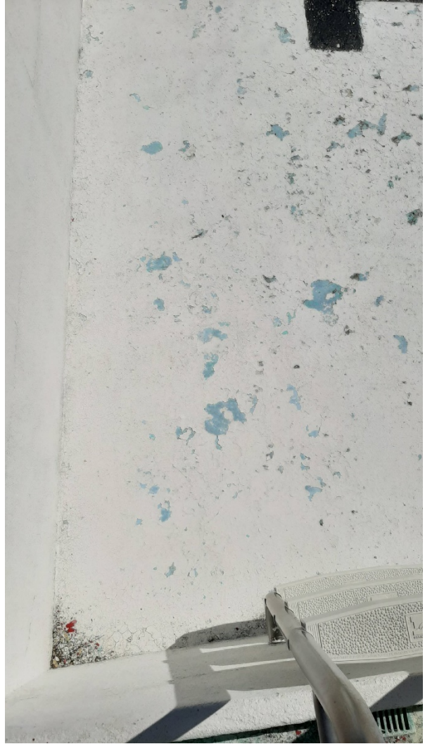
Figure 8. Eroding and chipped concrete prevents paint adherence (left); eroded concrete within pool (right)
