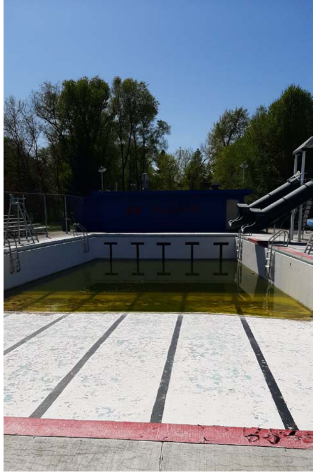
Figure 7. Shared office space/lifeguard area (top left), pool and deck edging showing visible wear/erosion (top right, bottom)
