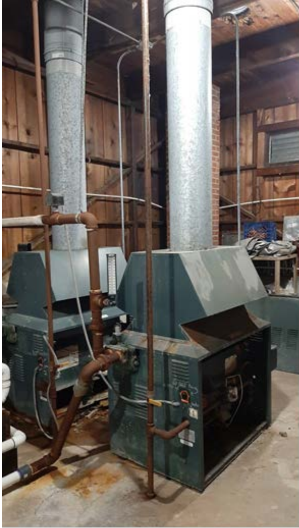
Figure 14. Pool boilers installed in 1990 (only one remains operable)
