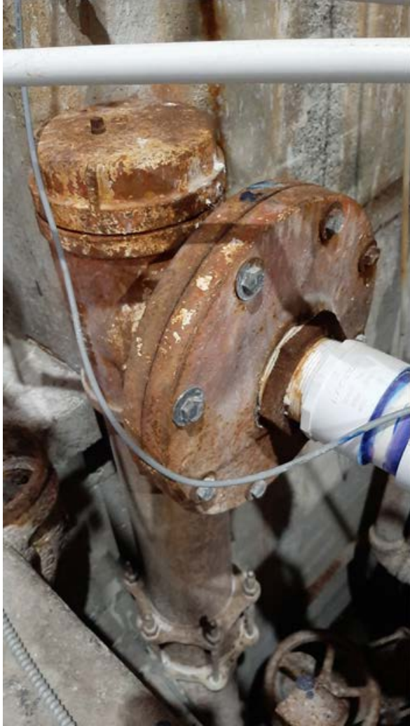
Figure 11. Galvanized pipe and casings (closeup)
