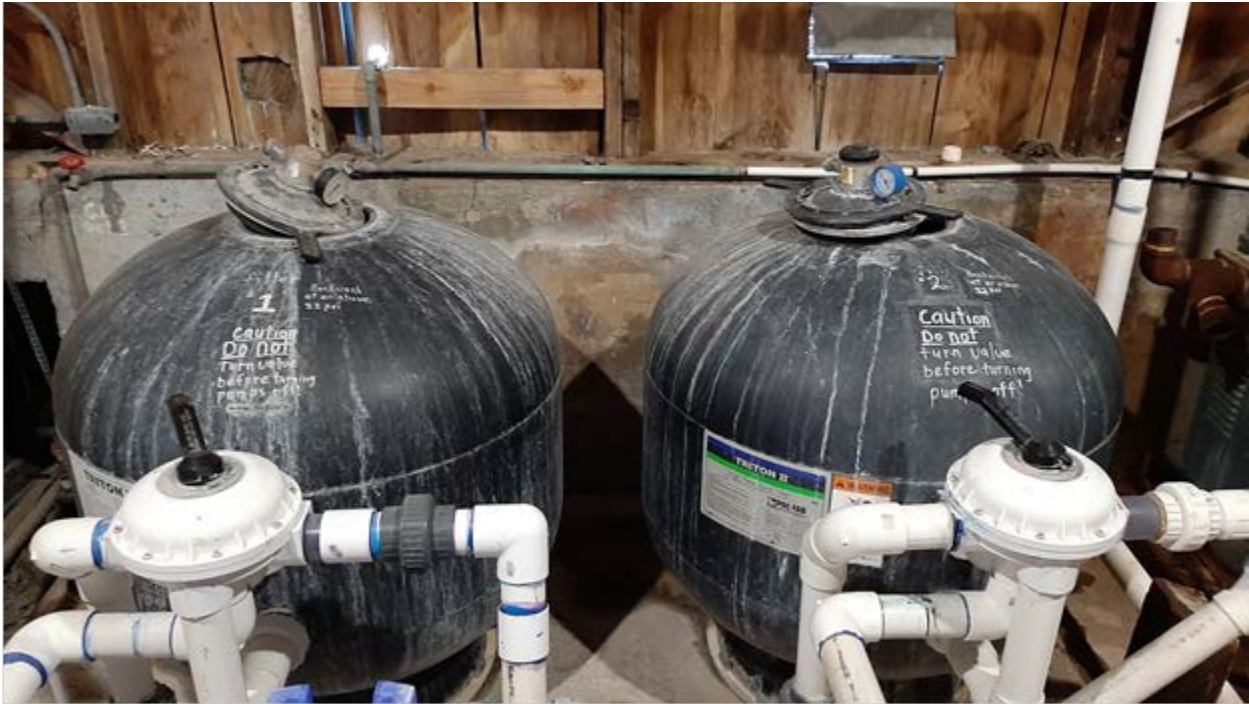
Figure 13. Dual sand filters
