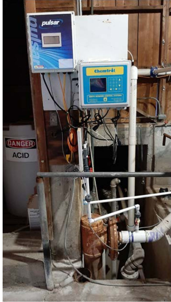
Figure 10. Corroded galvanized pipe and casings (left); chlorination system (right)
