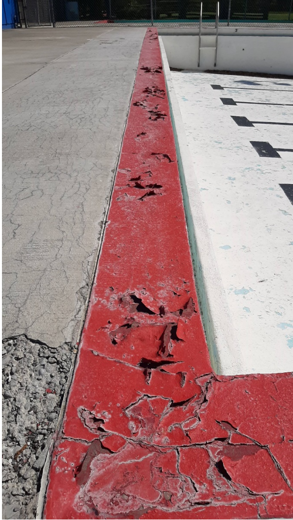
Figure 8. Eroding and chipped concrete prevents paint adherence (left); eroded concrete within pool (right)
