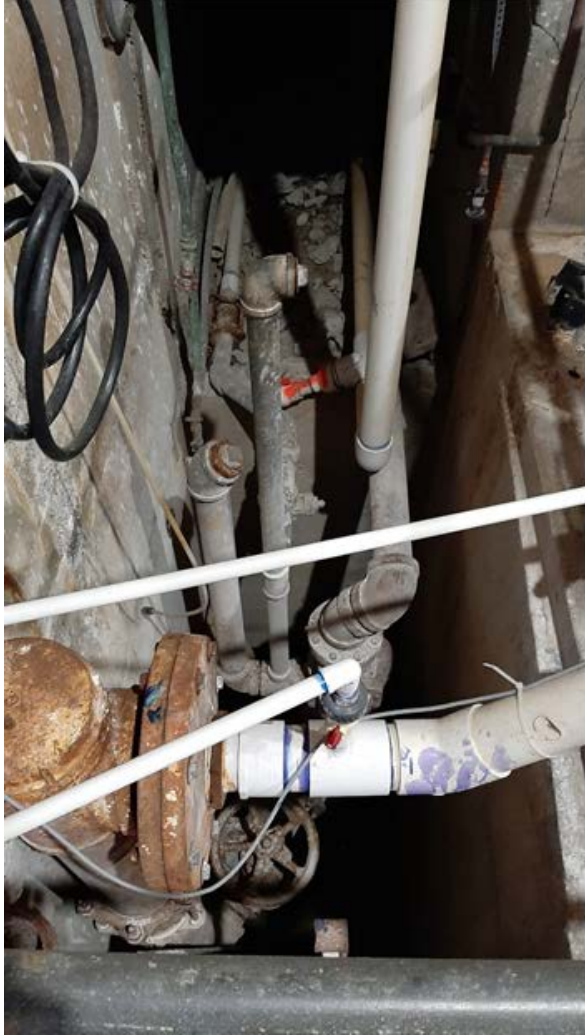
Figure 10. Corroded galvanized pipe and casings (left); chlorination system (right)
