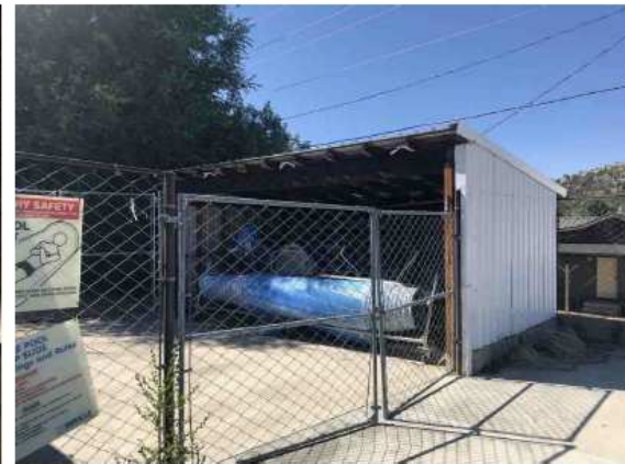
Pool Cover & Supplies Building
