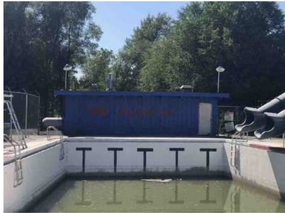
Pool Mechanical Building
