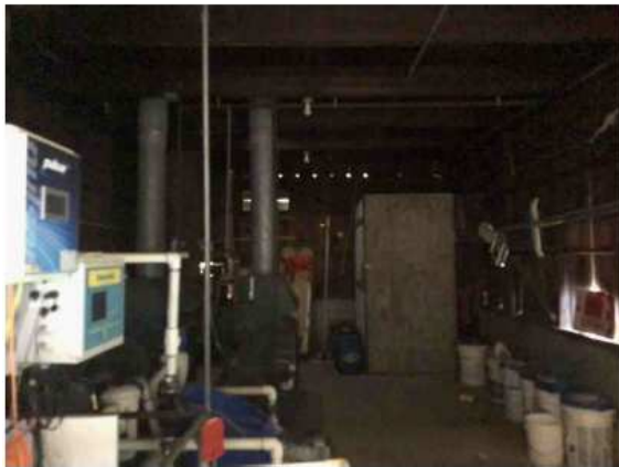
Interior of Mechanical Building
