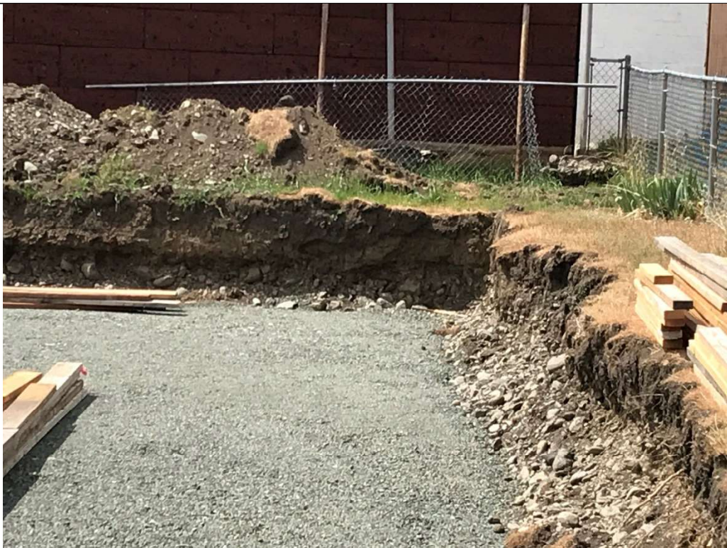
Photo 6. Close-up view of the home foundation excavation.
