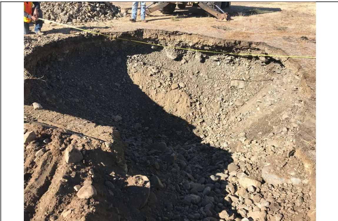
Photo 2. View of the completed test pit (looking north).
