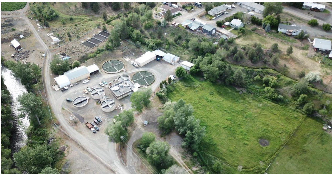
Figure 2. Current Wastewater Treatment Plant
