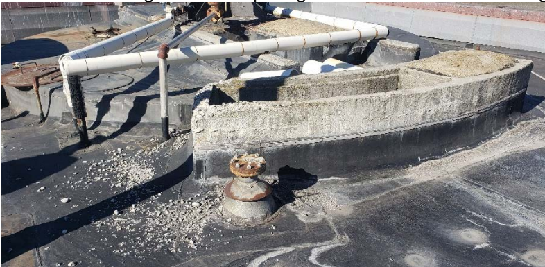
Photo 2 – Trickling Filter flow splitting structure – concrete cracking/weeping
