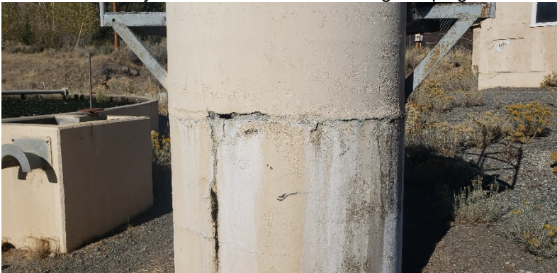
Photo 2 – Trickling Filter flow splitting structure – concrete cracking/weeping
