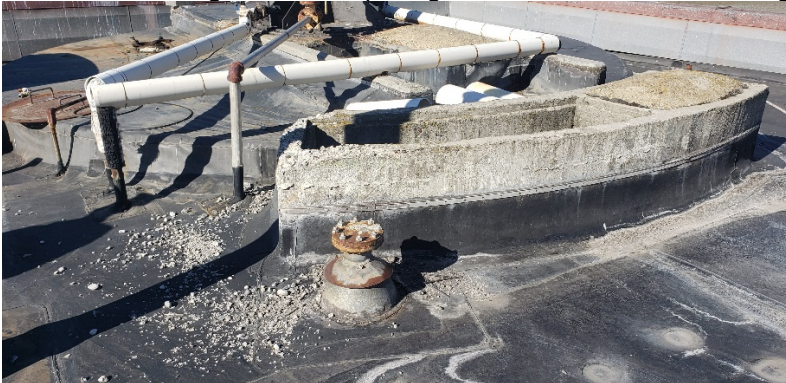
Photo 2 – Trickling Filter flow splitting structure – concrete cracking/weeping
