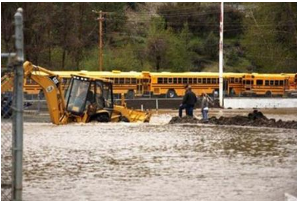
Figure 7. Flooding near John Day/Canyon City damaged the Grant-Union High School in 2010
