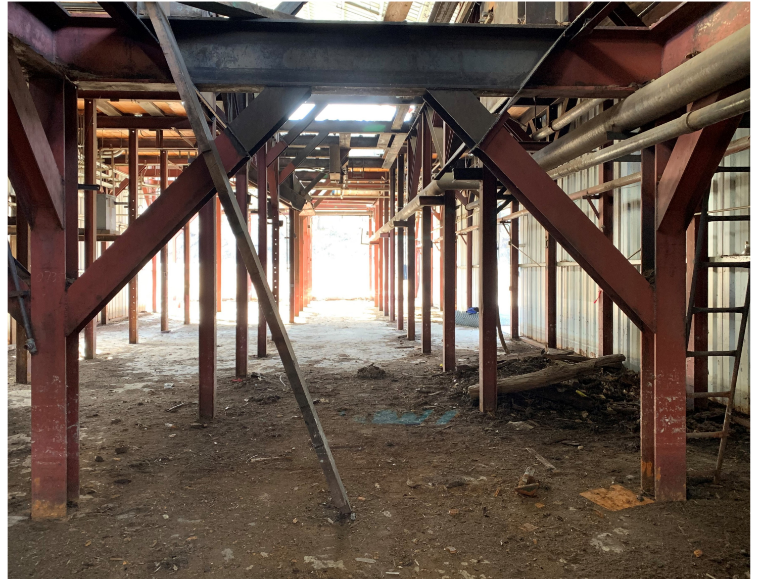
SAWMILL INTERIOR - LOWER LEVEL
