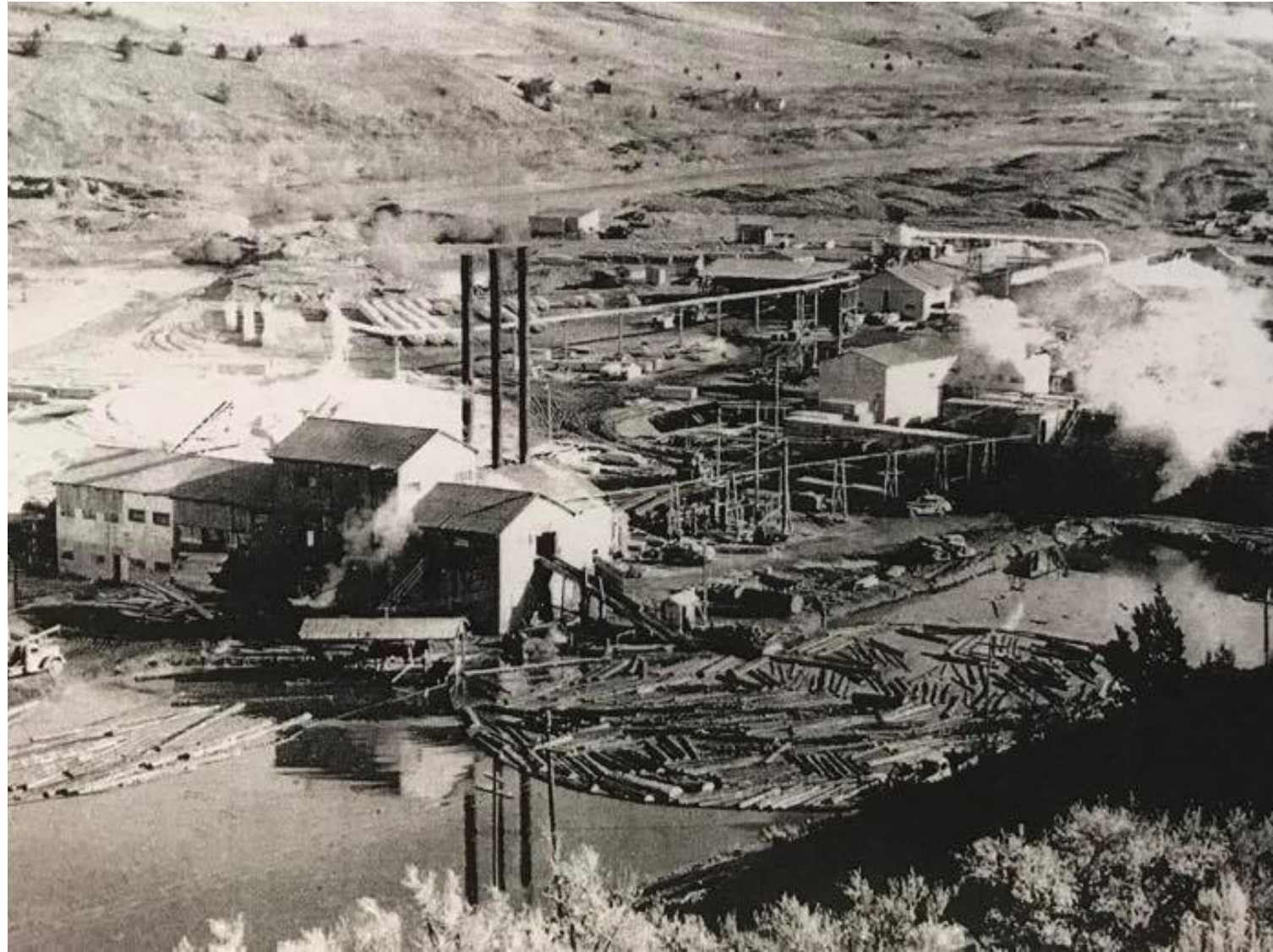
PROJECT SITE - BLUE MOUNTAIN MILLS - 1950s
