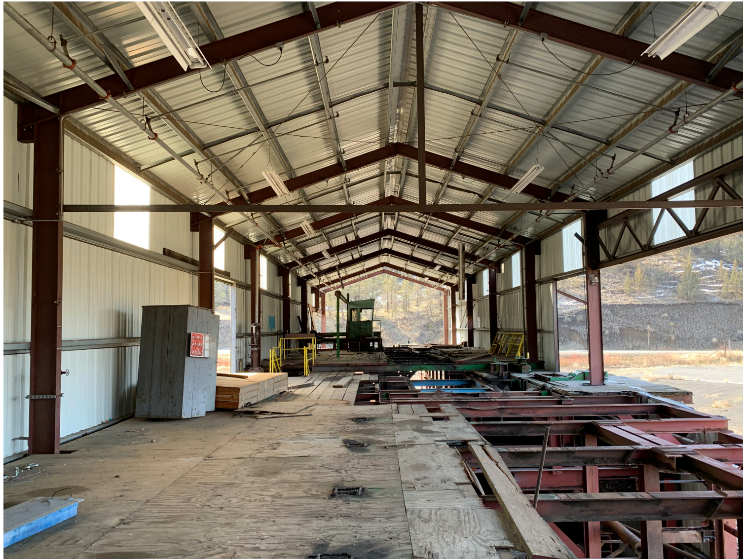
SAWMILL INTERIOR - MAIN LEVEL
