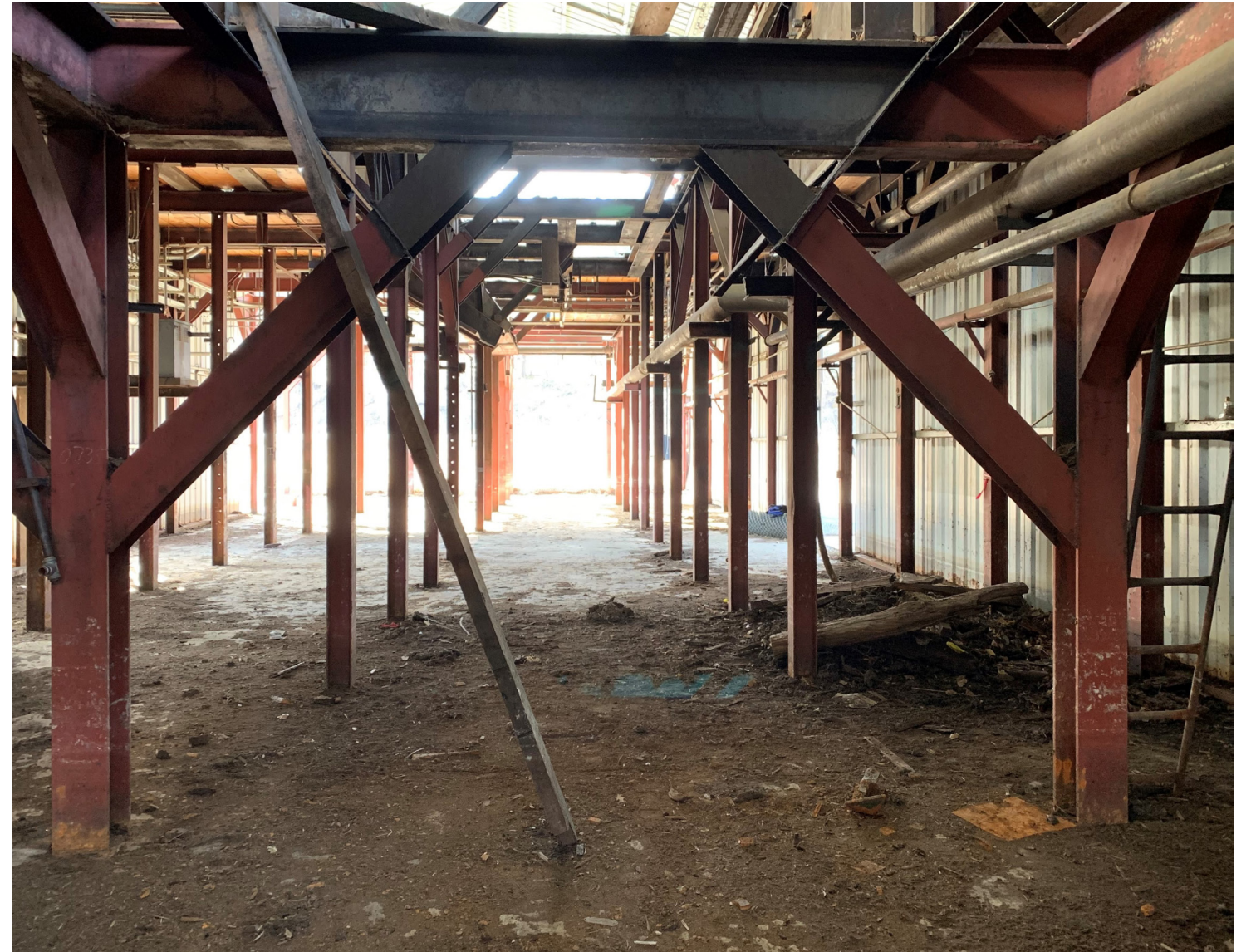
SAWMILL INTERIOR - LOWER LEVEL
