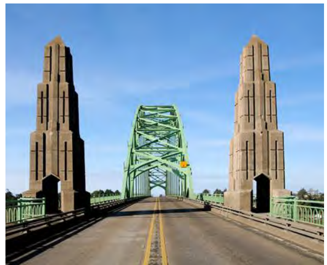
Many bridges on the Oregon Coast Highway 101 feature substantial vertical markers at each end
