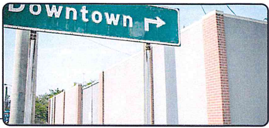
DECORATIVE RETAINING WALL
