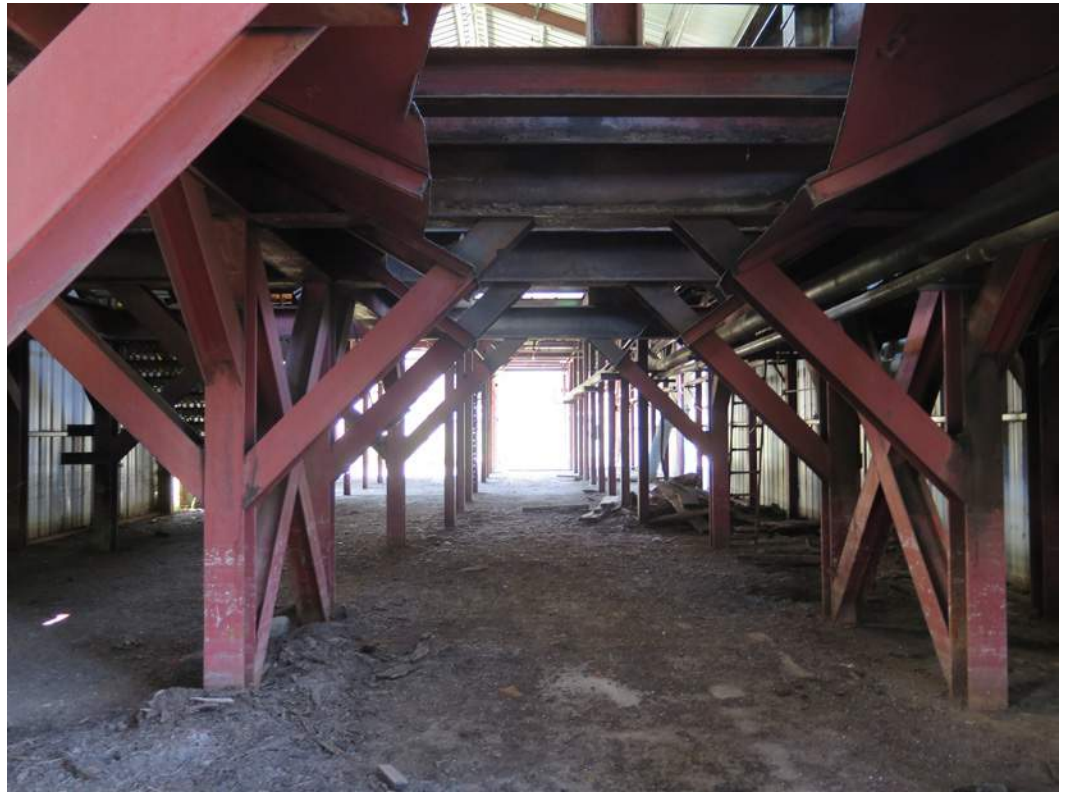
OREGON PINE: SAWMILL RESTORATION
