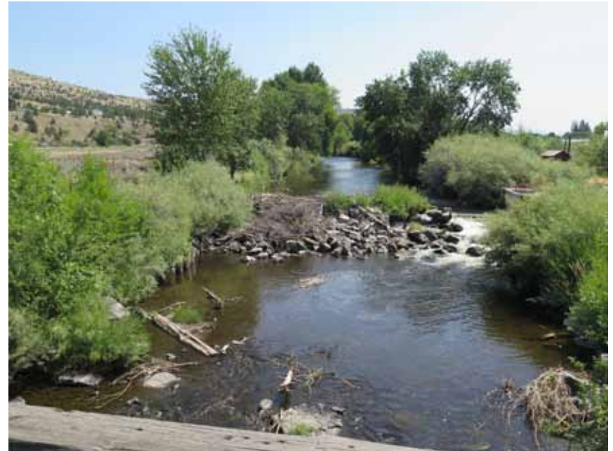
Irrigation diversion on Oregon Pine mill site
