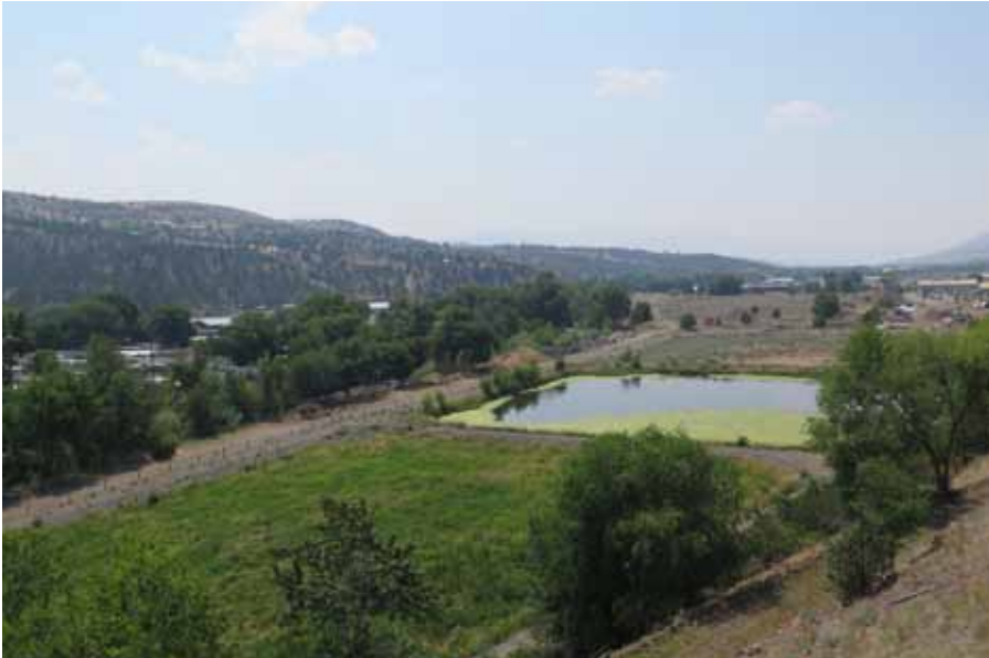
Current Wastewater Treatment Ponds
