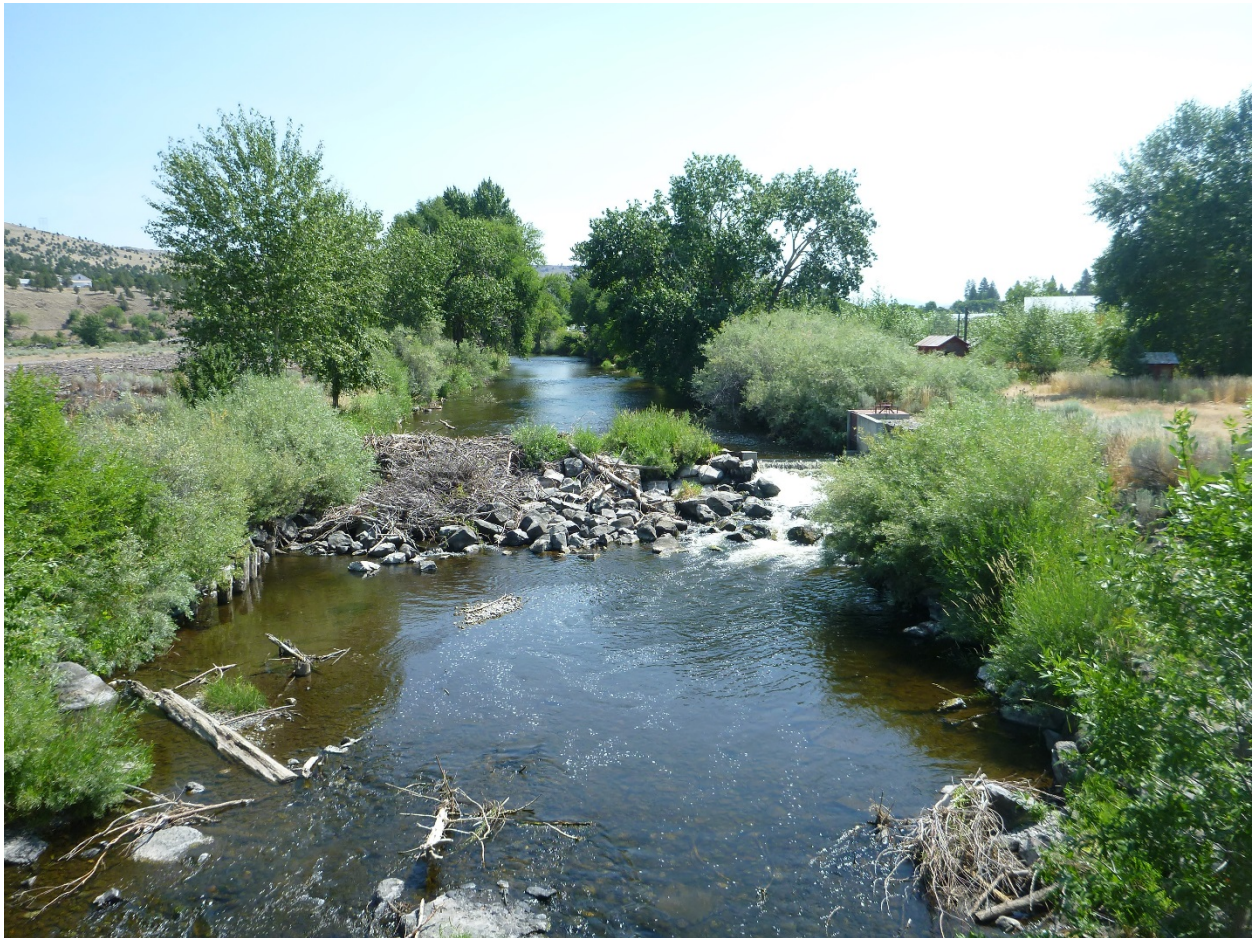
Figure 3.6. Low head boulder and concrete weir and irrigation diversion at downstream end of site.
