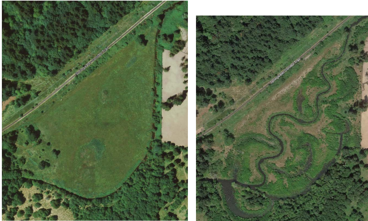
Figure 3.4. Aerial photos of the Johnson Creek Project, pre-project (left, 2006) and post-project (right, 2014).
