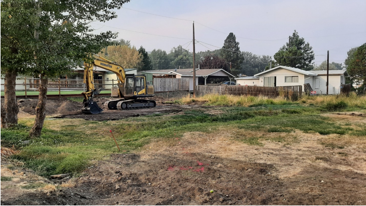
Figure 1. Trenching and Preliminary Grading, 7th Street Parking Area
