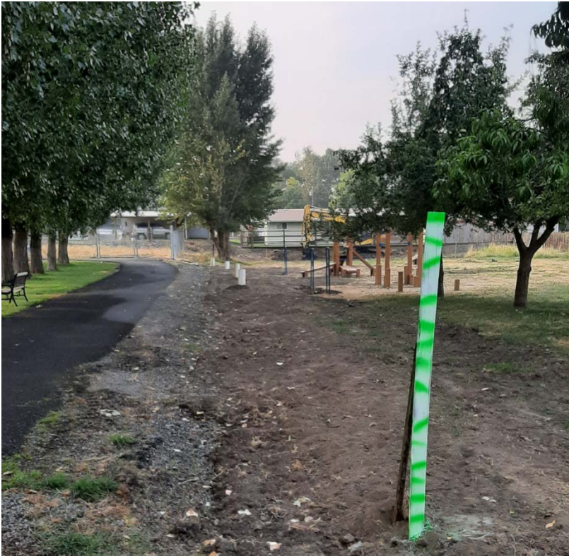
Figure 2. Utility trench for future electric and fiber conduit
